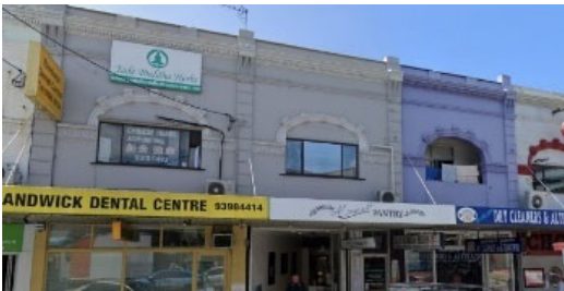
Figure 29: Inappropriate infill window / glazing framing
